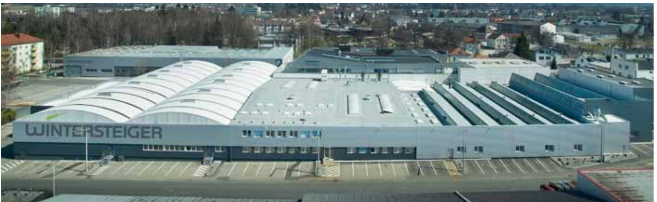
Headquarters located in Ried im Innkreis, Upper Austria
